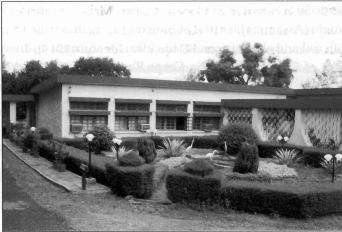
Fig.2. Laboratory building of Regional Station, Vittal
