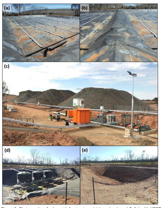
Figure 2: Photographs of relevant infrastructure: (a) heap leach pad Cell 1 with HDPE liner and drainage layer, (b) dividing embankment bund separating Cell 1 and Cell 2, (c) heap leach pad cells in operation, (d) PLS tank within HDPE-liner PLS pond, and (e) surface water management pond
