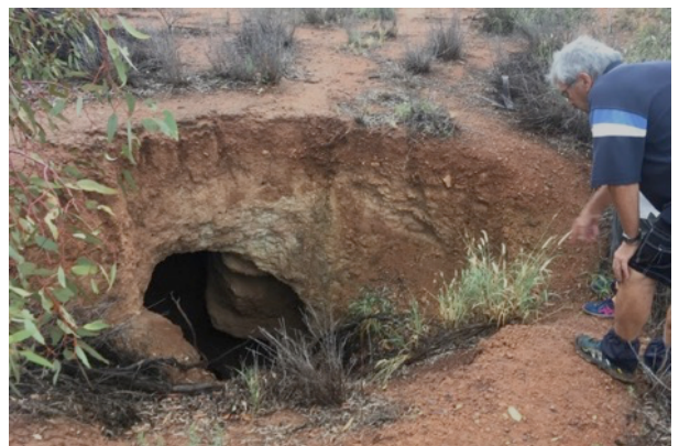
Neil and Connie inspecting the sinkhole at old Limestone Bore.
