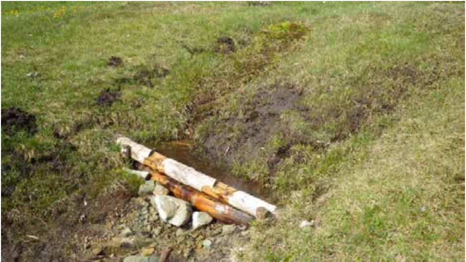
Photo 112: One of many dams constructed within the area occupied by flush fens in the Gorce National Park (photo by D. Horabik).
