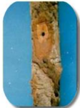
Bore hole damage
