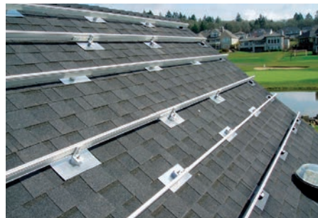
SHINGLE ROOF MOUNTING STRUCTURE FOR PITCHED ROOF
