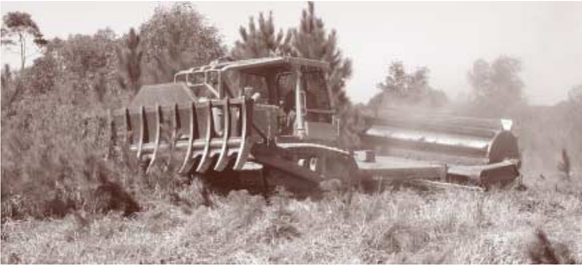
Site preparation in the Beerburum State Forest's Toorbul logging area. Strict controls ensure these sorts of activities impact minimally on the environment and include the use of specialised equipment such as this chopper roller.
