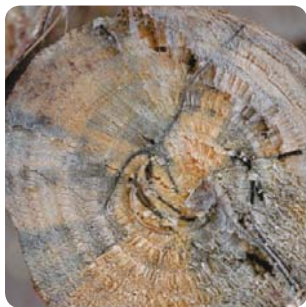
Timber staining caused by fungus (G Keith Douce)
