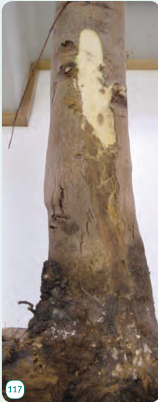
Cracking and cambial staining at base of E. dunnii following drought stress
