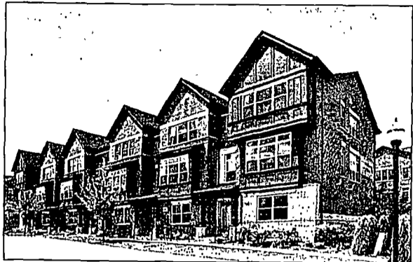
Jacobs Homes has opened another phase with newly reworked designs at Aspen Pointe, a community of 132 rowhomes set in Vernon Hills.
