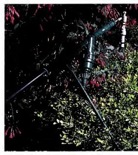
The "main assembly" consists of a metal atmospheric vacuum breaker to prevent dirt from getting siphoned into the home's water supply, a Yfilter and a water-pressure regulator.
