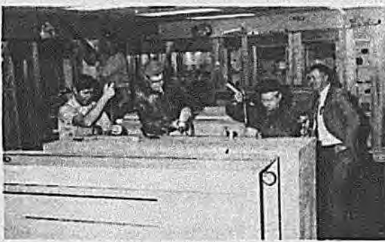
Nassau Carpenters Union workers in service on the renovation of the Heitz Place Courthouse, 1972.
