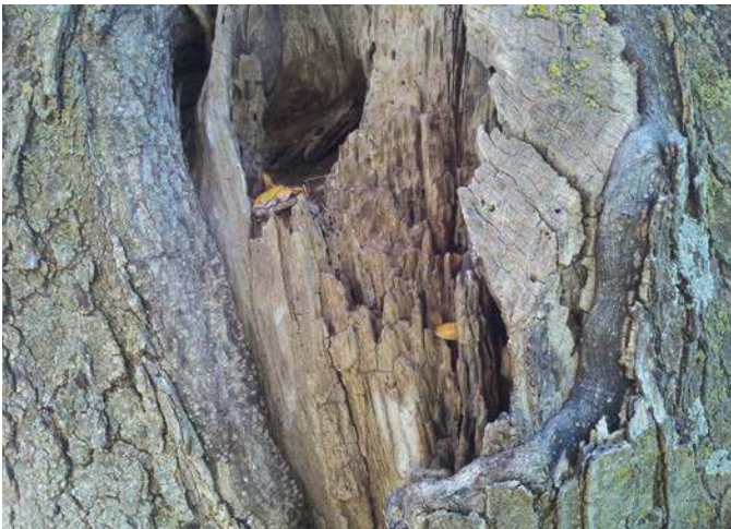
Photo 39. Crumbling wood indicates decay.
