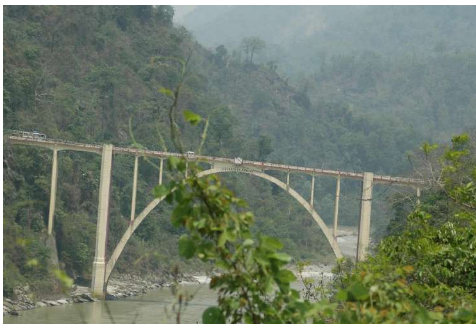
Upstream area of TLD Vth near Sevok Coronation bridge
