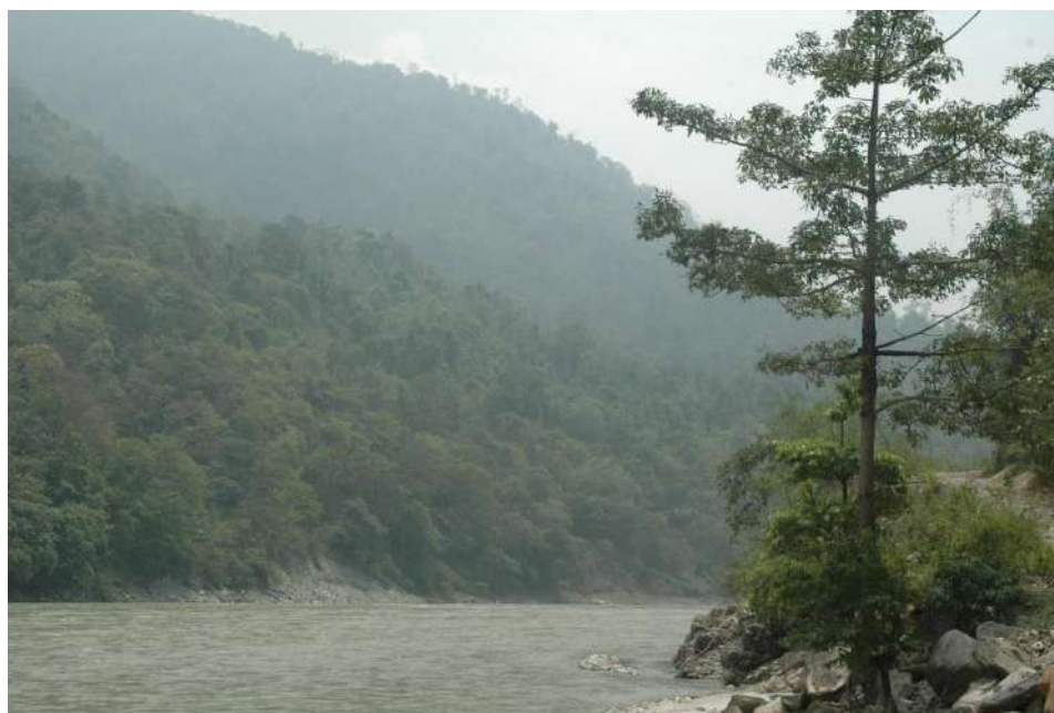
Dam site of Teesta Low Dam (TLD) IV project
