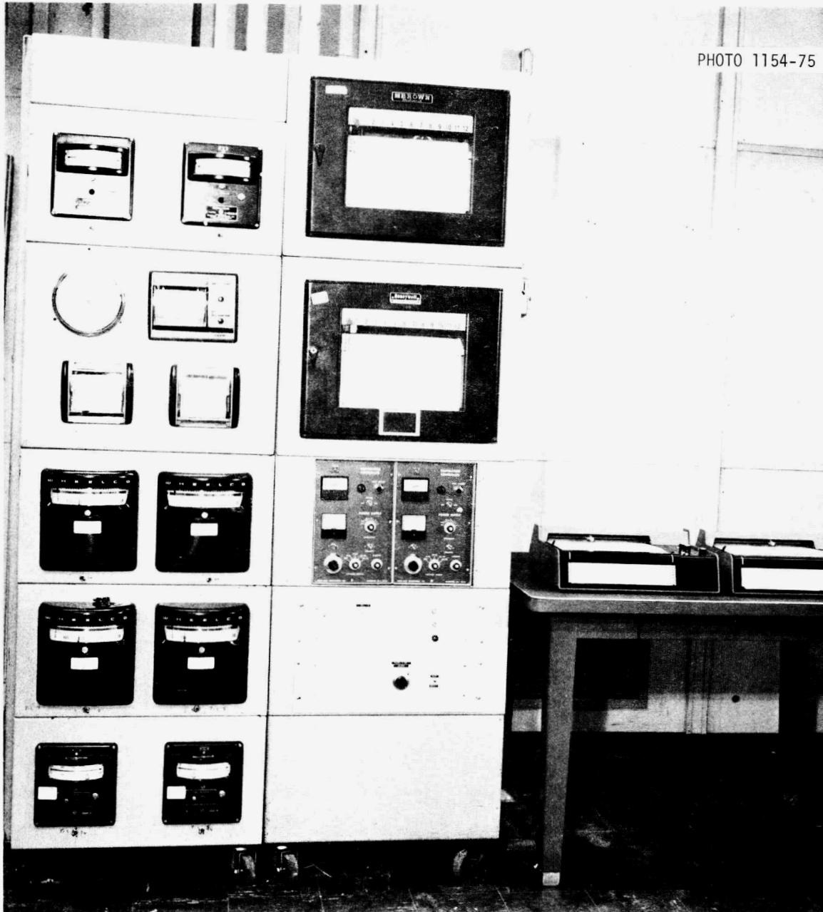
Fig. 16. Panelboard for Fuel Reconstitution Engineering Experiment temperature, level, and flow recorders and controllers.
