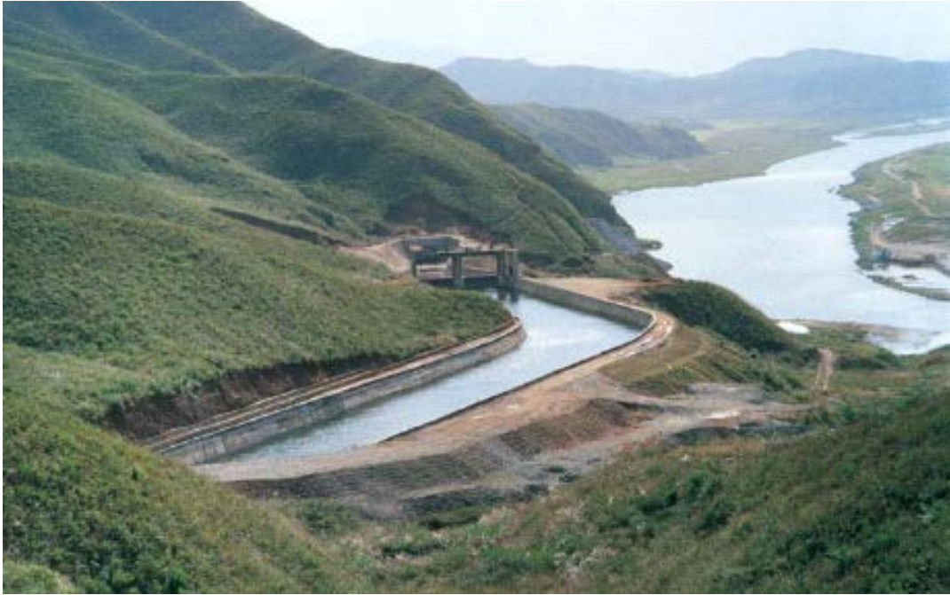
Figure 3-3: Recently-completed Natural-flow Irrigation Waterway in the DPRK 137
