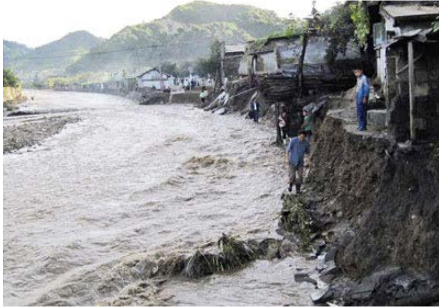
Figure 3-2: Flooding in Wonsan, DPRK in 2011 143
