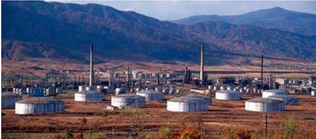
Figure 2-7: Photo of Sungri Chemical Plant Oil Refinery
