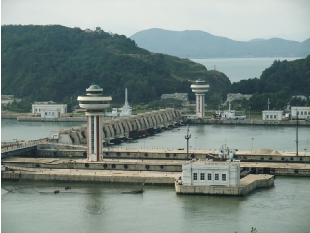
Figure 4-7: Photo of West Sea Barrage, Near Nampo, DPRK 213
