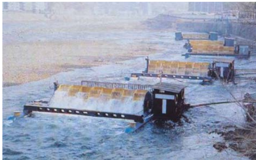
Figure 2-3: Photo of Kangae Hydro Power Plant 95
