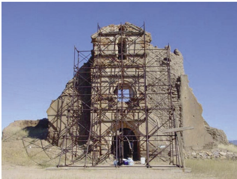
Fig. 7.10 The Nuestra Señora del Pilar y Santiago de Cocóspera mission at Sonora, México. The site represents a typical case where traditional restoration techniques proved detrimental to the preservation of the adobe bricks, requiring new consolidation materials to be developed. Reprinted with permission from reference number [71], Copyright, Elsevier Ltd
