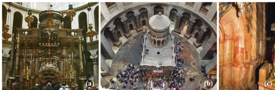
Fig. 5.15 Image of the Holy Aedicule before interventions: front view (a), top view (b); intense buckling of the structure (c)
