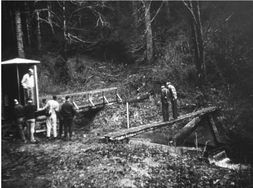
Fig. 2.5 Broad crested compound V-notch weir on Deer Creek
