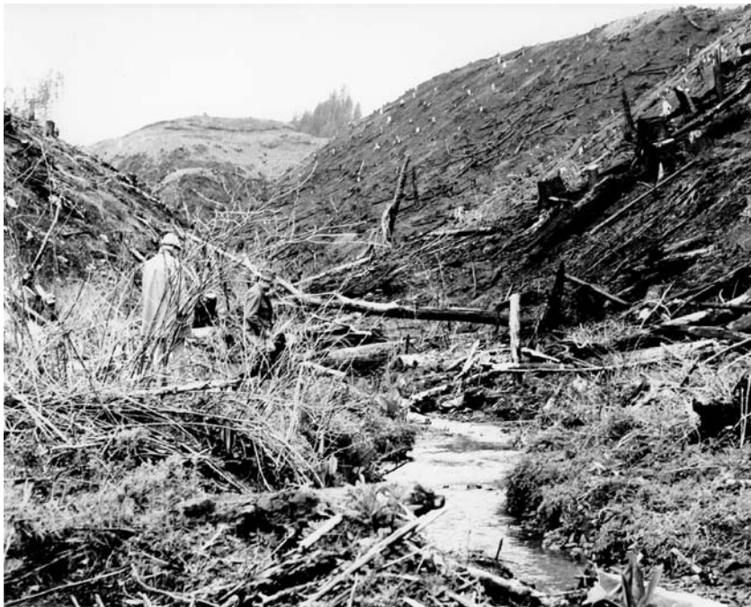
Fig. 5.4 Looking upstream into the canyon of Needle Branch at approximately 500 m above the fish trap during winter 1966–1967, after stream clearance and the slash fire
