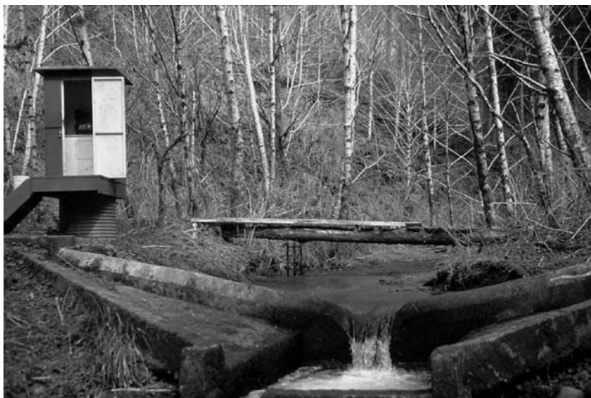
Fig. 1.4 Broad-crested compound concrete weir with stilling well on Flynn Creek
