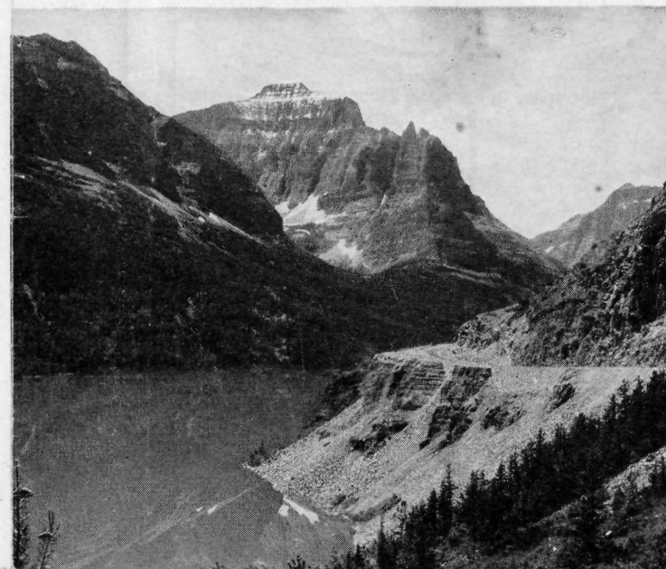
St. Mary Lake, Little Chief Mountain, and Going-to-the-Sun Highway (Hileman Photo)
