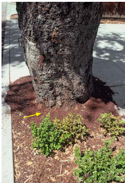
Figure 7.18. A large quantity of frass (fecal pellets and boring dust) has accumulated around this oak (arrow), indicating an infestation of carpenterworm ( Prionoxystus robiniae ). Root injury due to sidewalk repair likely predisposed the tree to infestation. B. HAGEN
