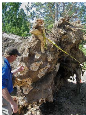
Figure 7.137. Although this large coast live oak appeared relatively healthy before it failed, nearly all of the large supporting roots were decayed by oak root fungus ( Armillaria mellea ). T. YOUNG
