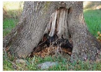
Figure 7.146. Cavity and basal decay resulting from fire damage to the lower stem of a valley oak. B. HAGEN
