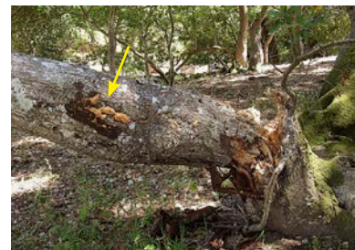
Figure 7.122. Oaks killed by sudden oak death ( Phytophthora ramorum ) are prone to rapid wood decay and structural failure. This coast live oak failed less than a year after it was killed by the disease. Fruiting bodies of a wood decay fungus (probably Phellinus gilvus ) can be seen growing on the trunk. B. HAGEN
