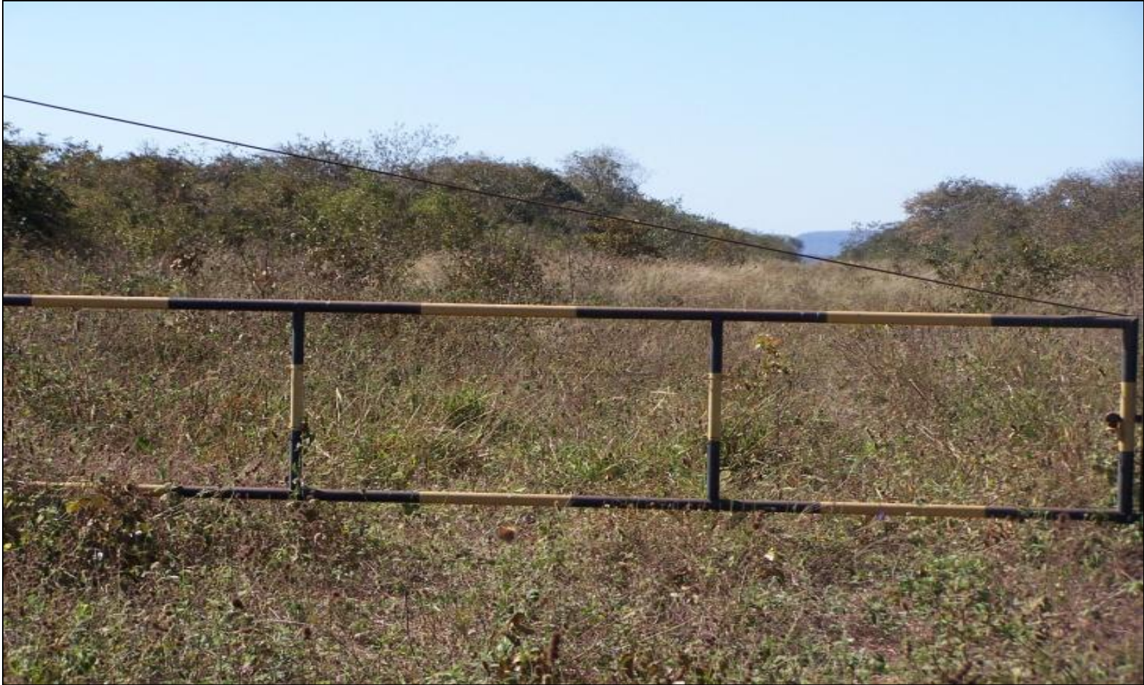
Figure 14. Portion of the Bolivia-Brazil pipeline in Santa Ana de Chiquitos (July 2008).
