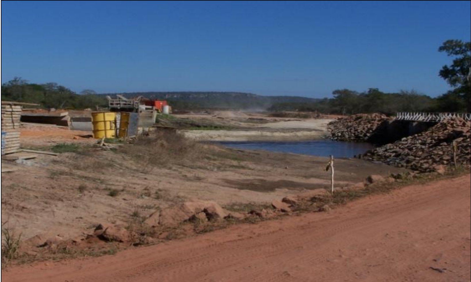
Figure 13. Challenges with constructing a bridge over the Rio Quimome (July 2008).
