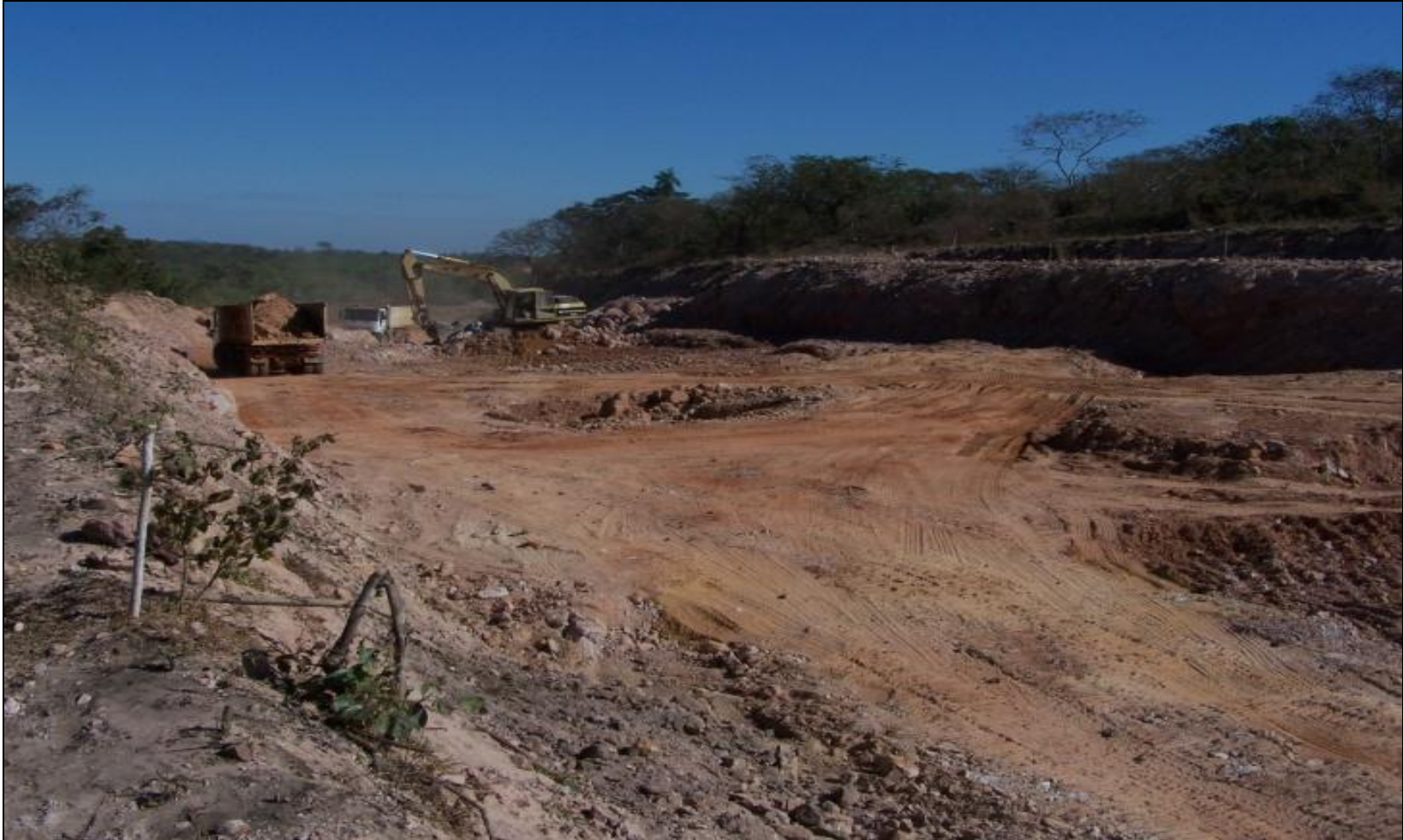
Figure 12. New highway construction between El Tinto and Quimome (July 2008).
