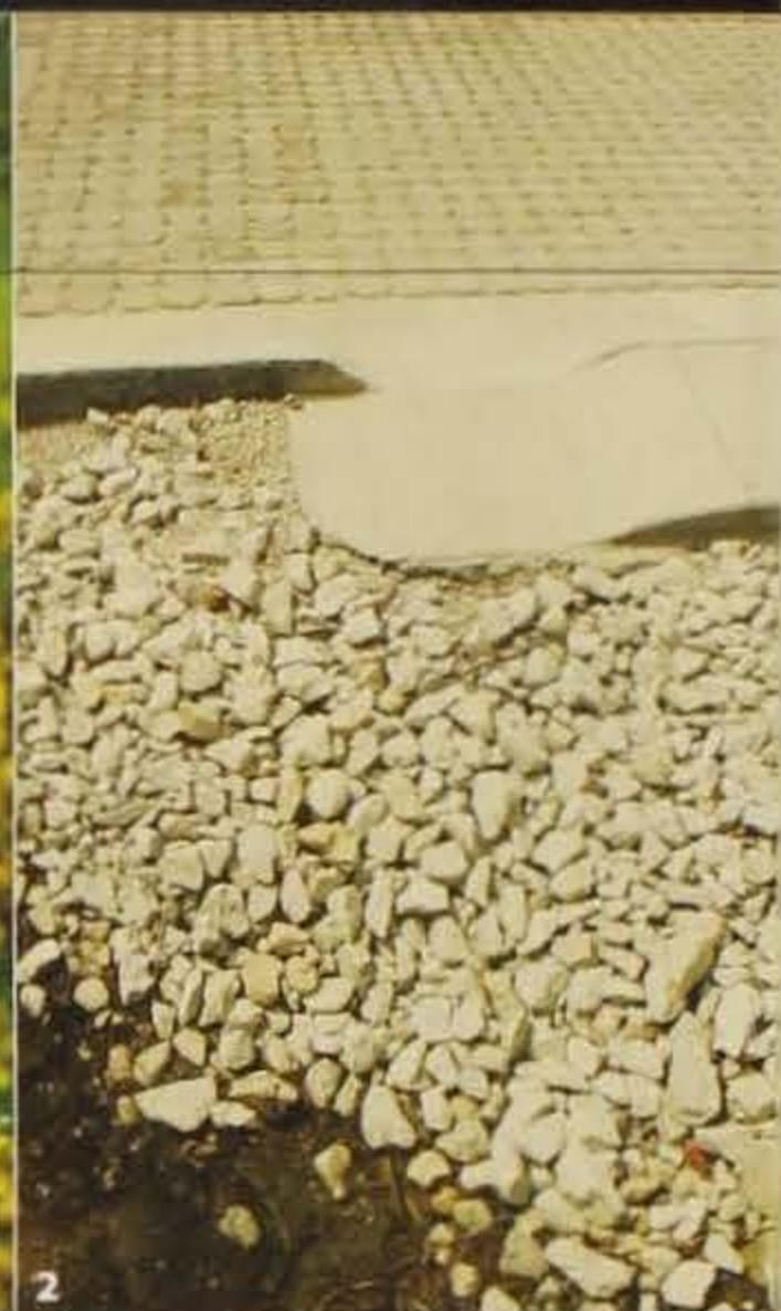
1) Rose mallow ( Hibiscus laevis ) adds distinctive flower shape to gardens. A lover of wet ground, it may reach 6 feet heights, so allow plenty of space. 2) Roof runoff flows across porous pavement that allows water to enter the soil with excess flowing toward an adjacent rain garden. 3) Droplets splash onto a permeable parking area to absorb into the ground, reducing flow to city storm drains. 4) Late season color. 5) Black-eyed susan. 6) Fluted, colorful red cardinal flower will attract hummingbirds. FACING PAGE: Oil-laden runoff flows between parking lot curbs towards bed of sneezeweed.
