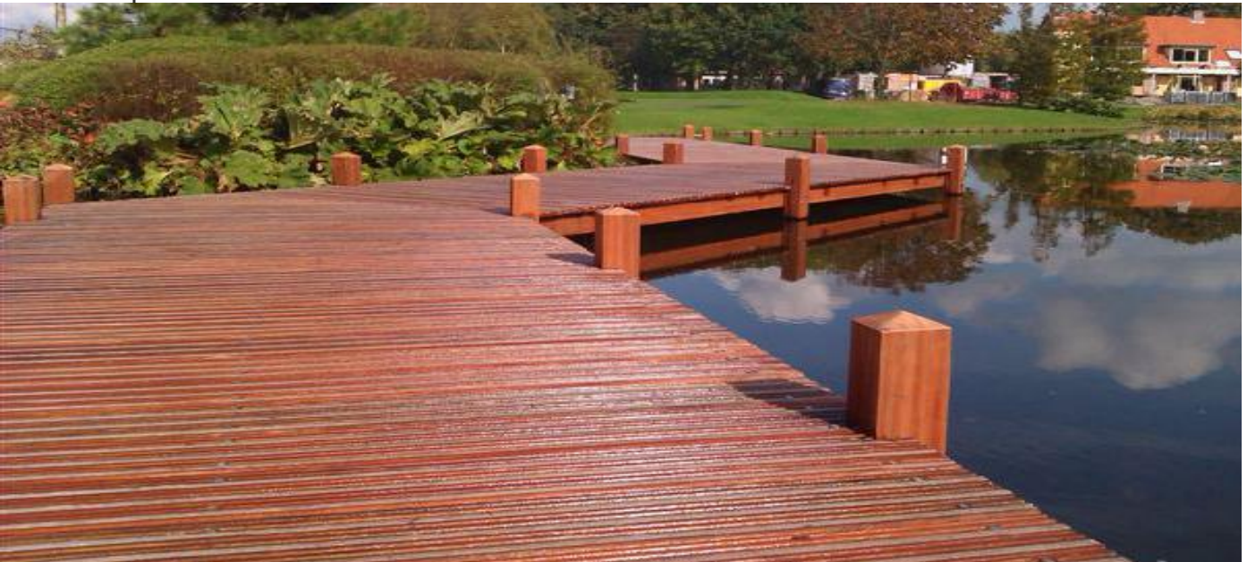
Bridge with Cow Wood/ Tatajuba decking and beams.
