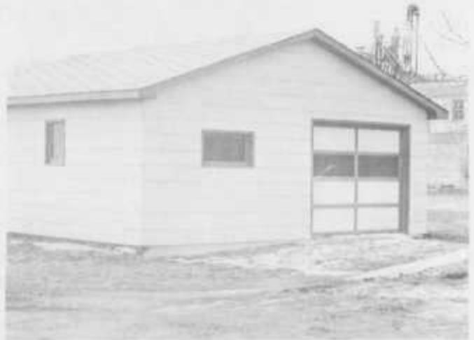
Park Board Committee, Park concession stand built 1980
