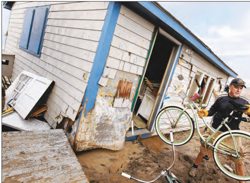
Pete Duhamel, of South Kingstown, R.I., removes a bicycle from a cottage Tuesday while helping a friend salvage belongings from the structure destroyed by Sandy, on Roy Carpenter’s Beach, in the village of Matunuck in South Kingstown.
