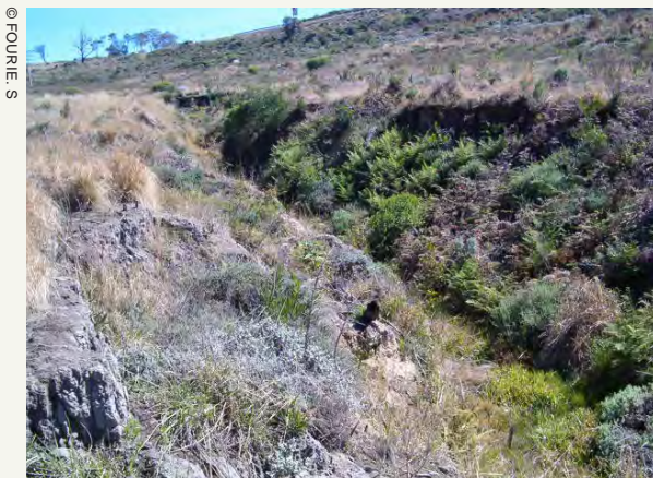
An example of bank slumping in the pictures after clearing of IAPs, with re-adjustment of slope and establishment of indigenous vegetation. The picture shows an example of an area with a lower gradient below an invaded and incised channel, where sediment is being trapped. Cynodon and Kikuyu have established on this site.
