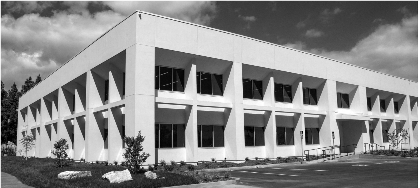
City-owned building located at 12616 183rd Street
