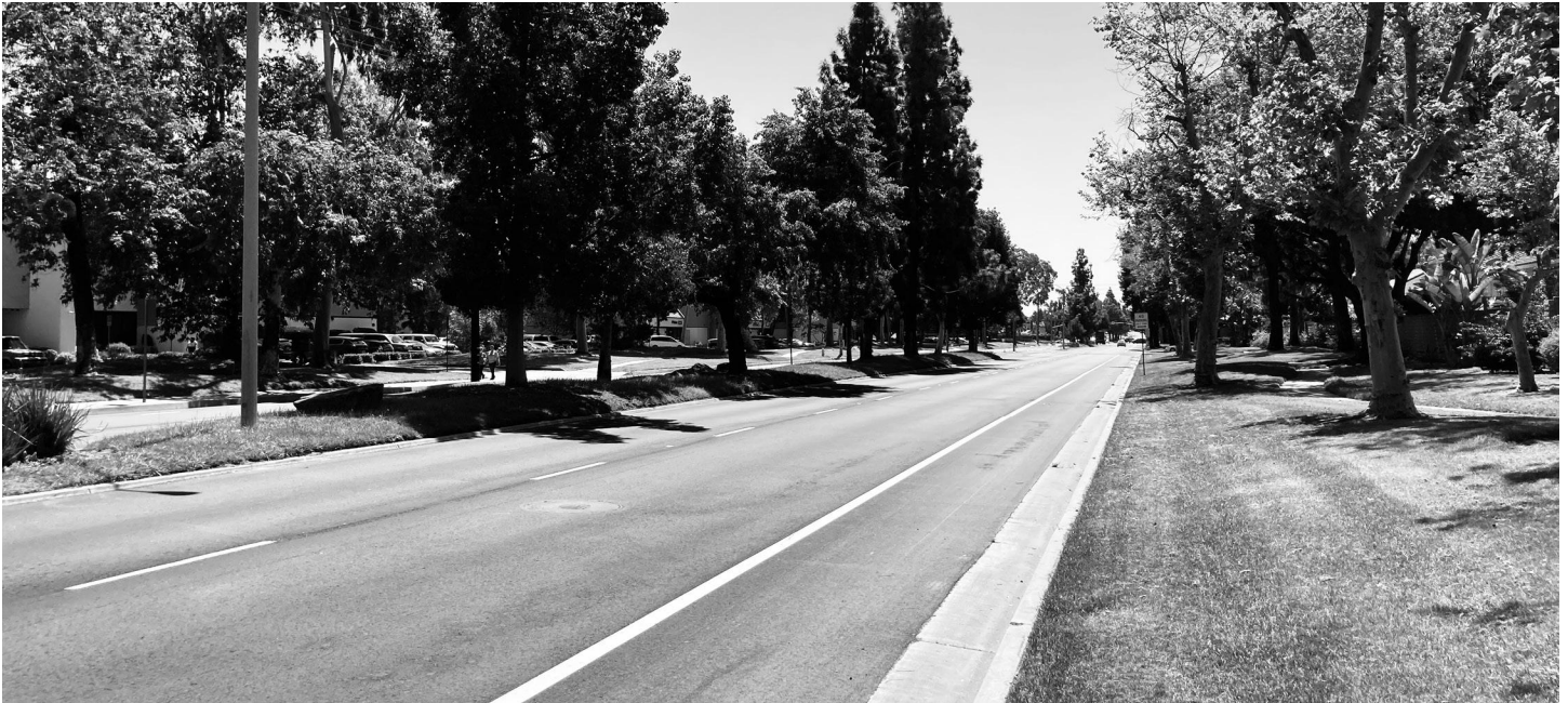
Bloomfield Avenue Street Improvements
