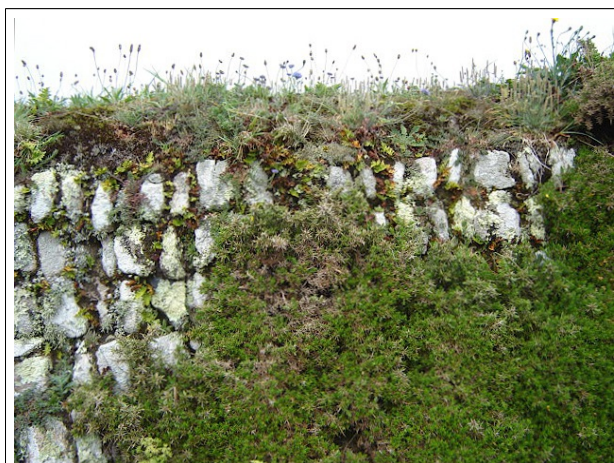
This beautiful old Cornish hedge near Cape Cornwall, built by a master craftsman and encrusted with many lichens, mosses and small ferns, is being destroyed by a thick mat of gorse as the flail forces it to spread across the face of the stones. This eliminates the lichens and in time loosens and dislodges the stones.
