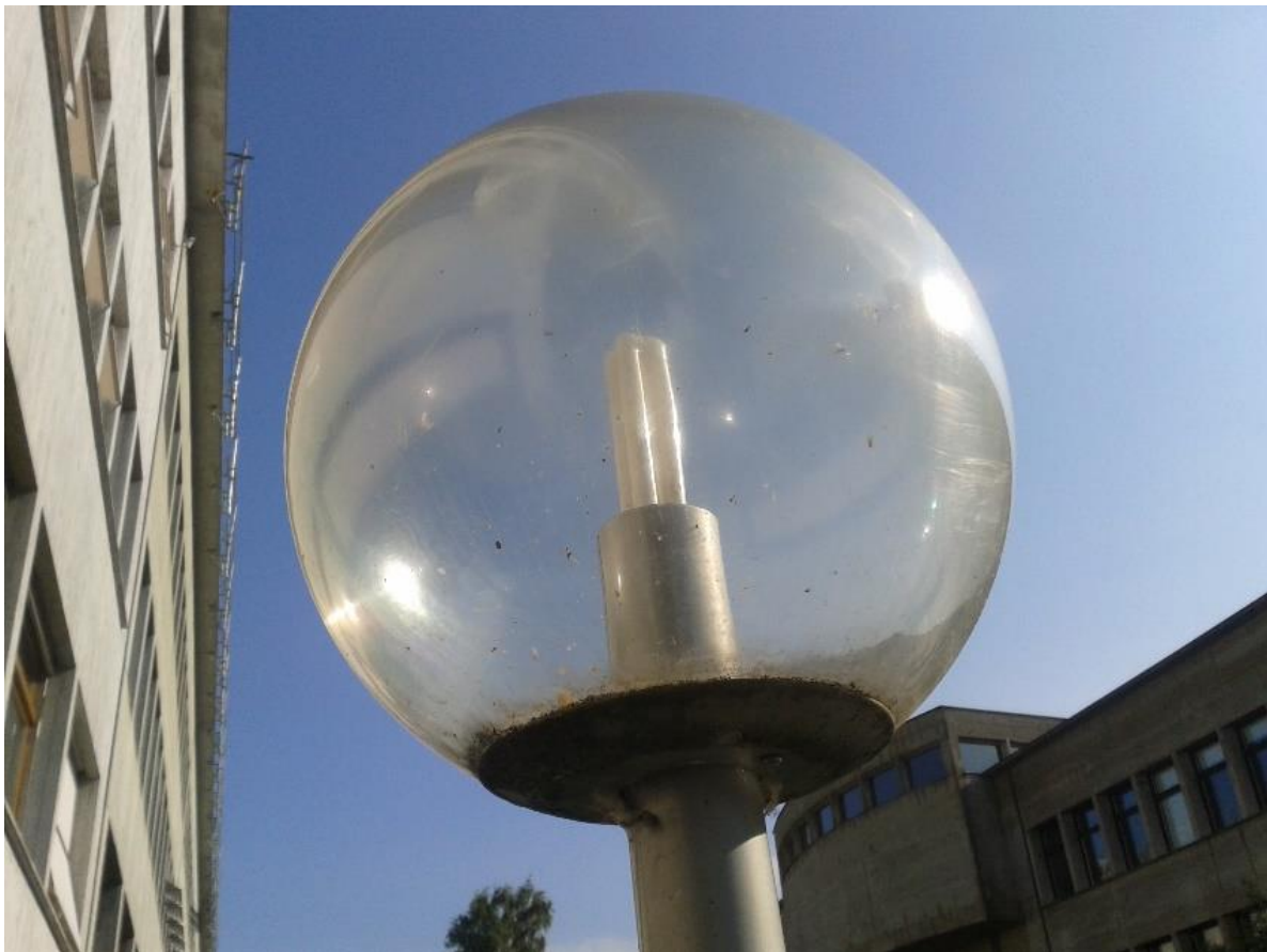
Fig.7 An illustration of why comprehensive data on outdoor lighting is needed. In this case, simply recording the bulb type (energy efficient compact fluorescent) gives no indication that it is fitted into a highly inefficient lamp design (lacking any shielding to restrict up-lighting).
