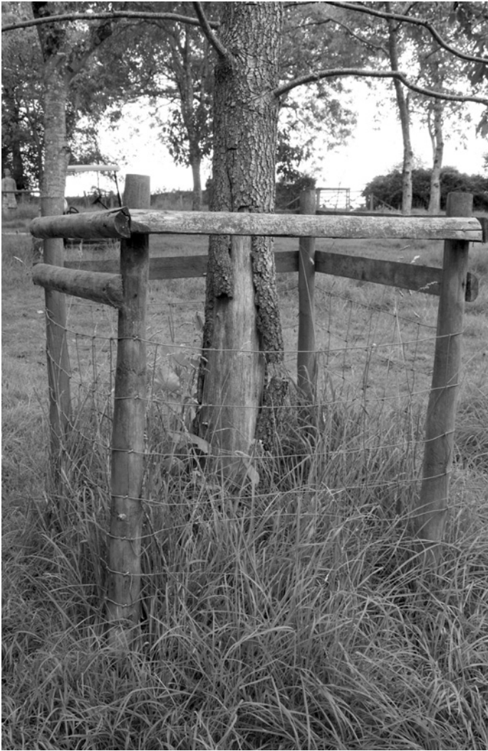
Damage as a result of the freeze
