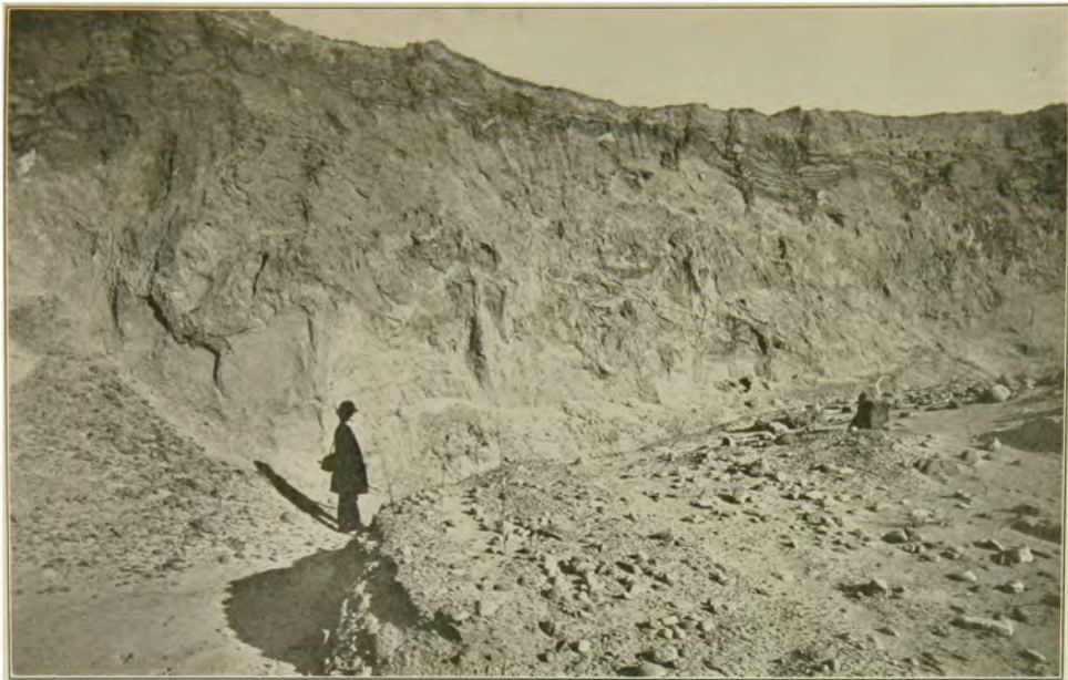
SECTION AT SOUTH CLINTON STREET Excavation west of the street. Looking southeast. Sands highly crumpled
