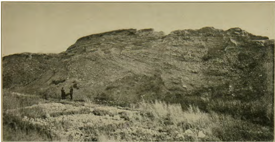
GRAVEL EXCAVATION SOUTH OF BRIGHTON East side of Winton Road. Duffy pit. Looking southeast
