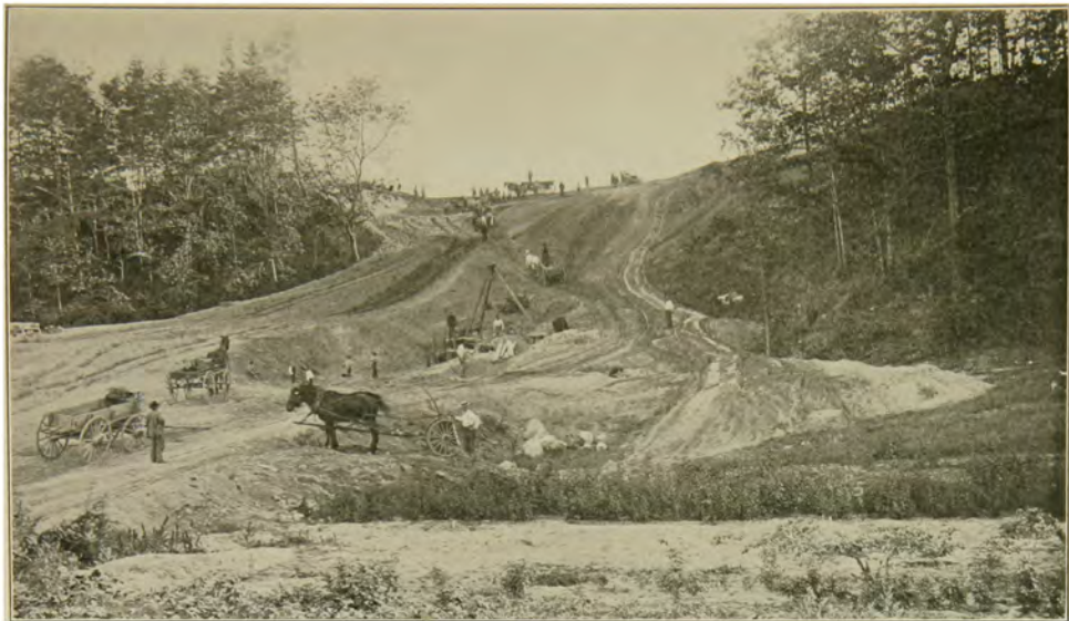
SOUTH GOODMAN STREET SECTION Cutting for street extension. View looking south
