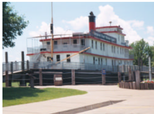
National Park Service photo
