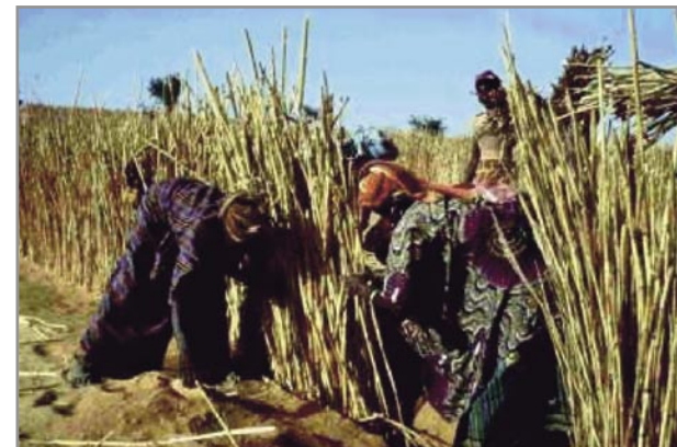
Niger. Dune fixation under the Keita (funded by Italian Government) project. Dune fences are made from dried millet stalks.. Photo: F. Paladini FAO/15337.
