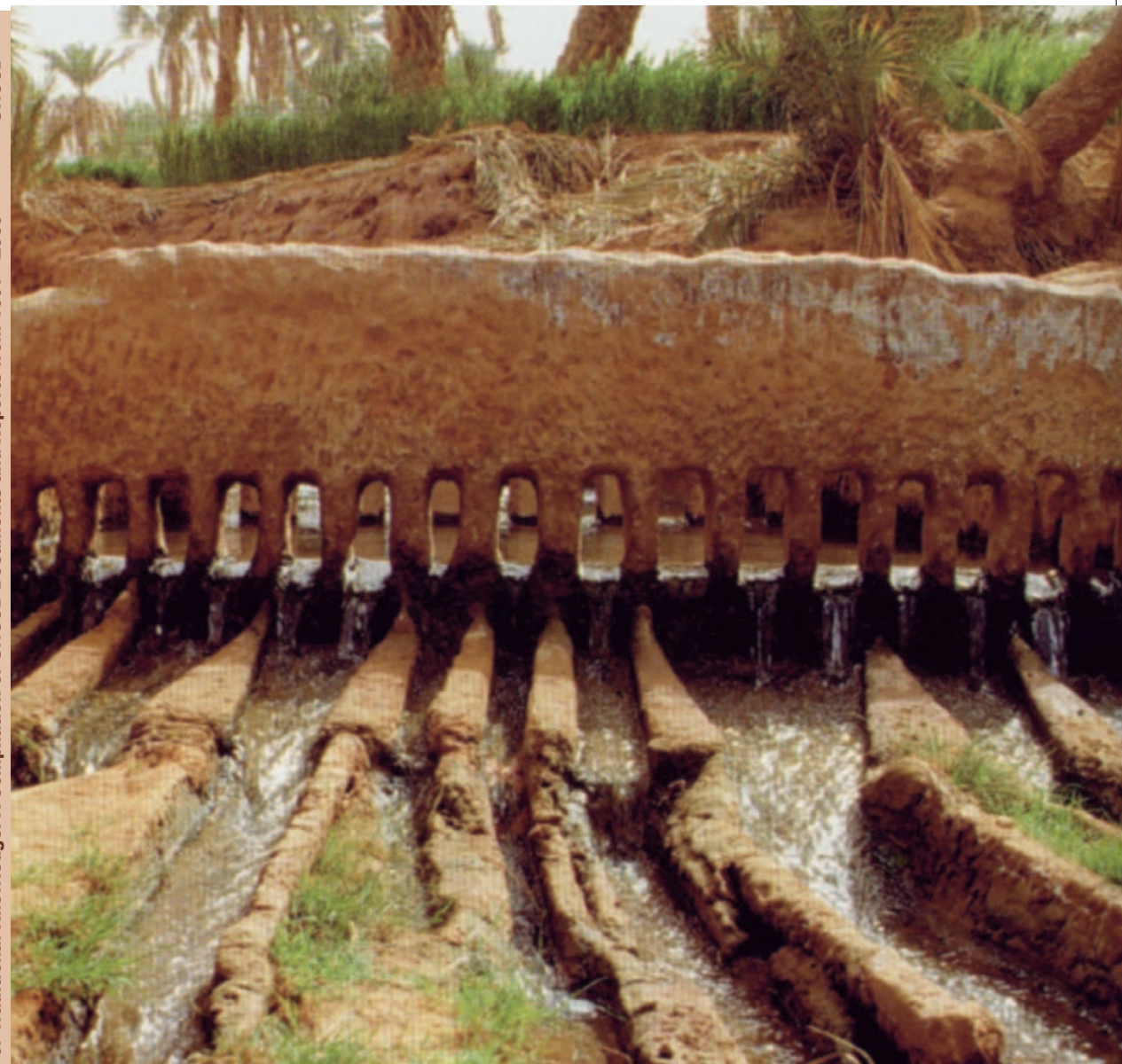
Oasis of Timimoun (Algerian Sahara), kesria, a water quota sharing system. Photo: P. Laureano.
