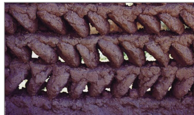
The adobe walls surround the small tilled parcels and contribute to the water balance. When the wind penetrates the narrow interstices in the plano-convex bricks it accelerates and expands making the temperature decrease. The raw earth mixture absorbs and releases humidity into the soil. Photo: P. Laureano.
