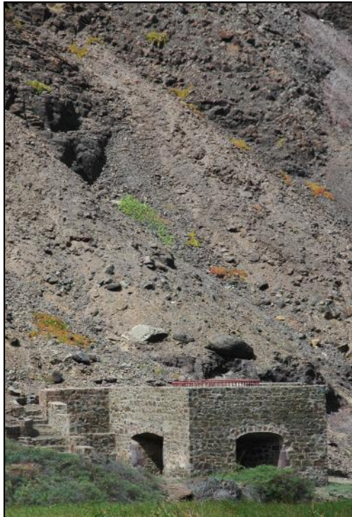
Figure 12: Restored in 2001, this is the lime kiln used by the East India Company.
