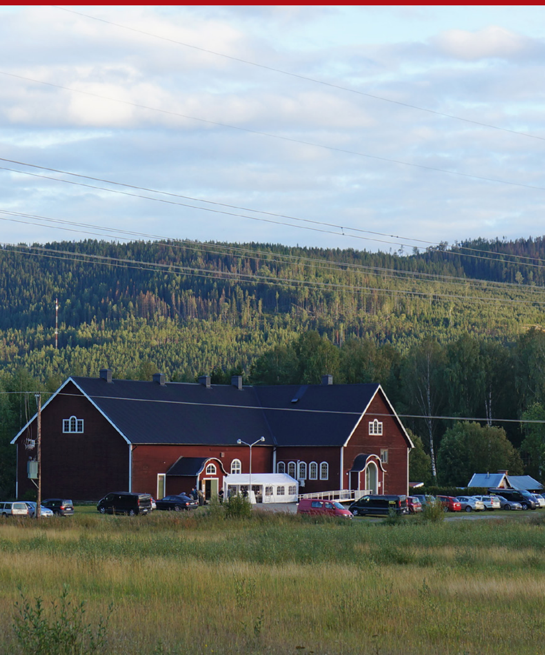
Erikslunds Folkets Hus, our working site. Photo: Olga Morozova
