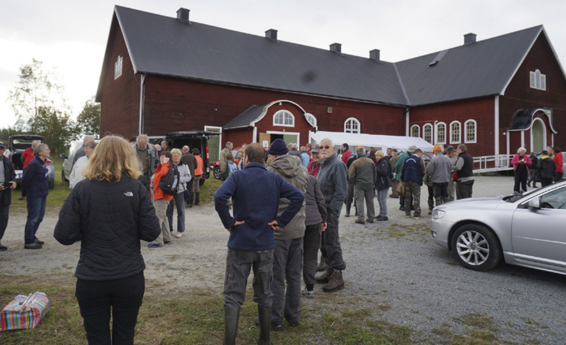
Erikslunds Folkets Hus, our working site. Photo: Olga Morozova
