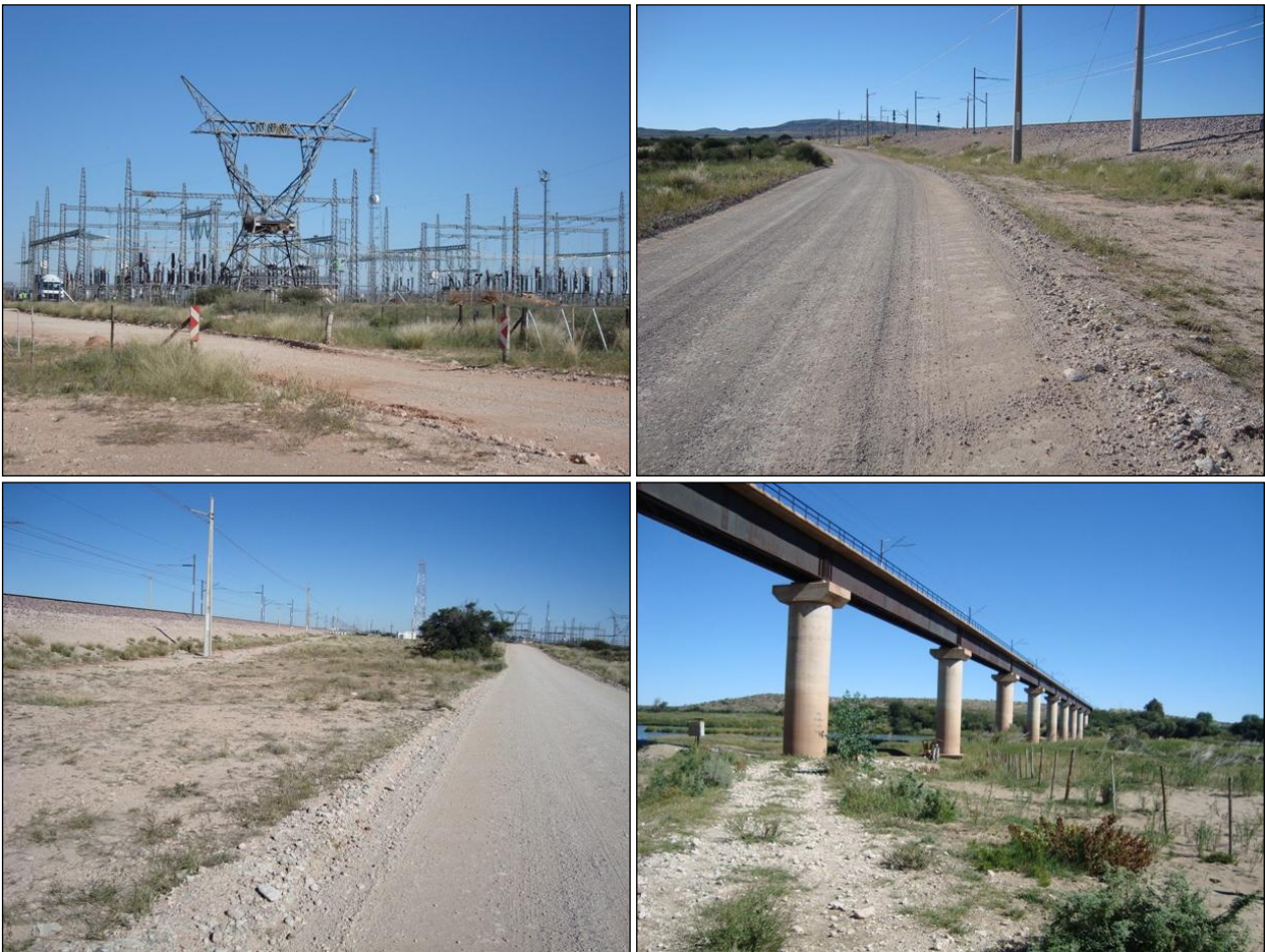
Figure 1: Various views of impacting features associated with the proposed pipeline alignment route.
