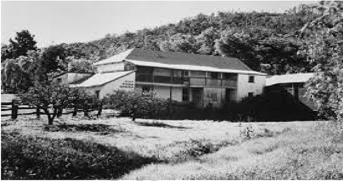
Figure 7-2 Whitby Falls Hostel (Conservation Plan, Griffiths Architects 2013)
