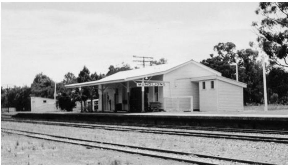
Figure 7-3 Mundijong Station (#19 on the Heritage List) (J. Austin, railheritagewa.org )
