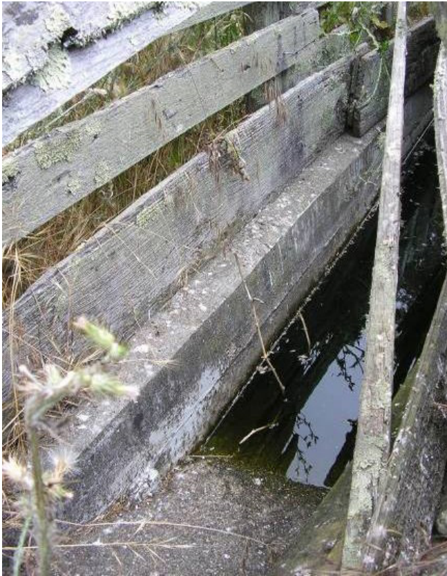
Waste disposal site in gully
