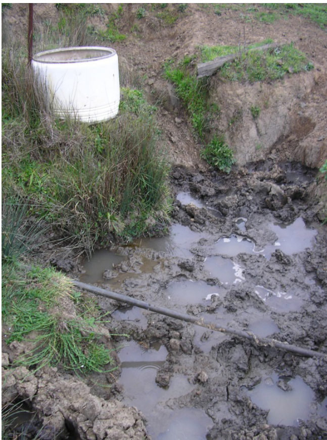
Spring requiring repairs
