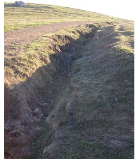
Photopoint 92. Erosion along road.
