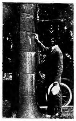
FIG. 50. - Concrete filling built in sections. (From "Tree Talk.")
