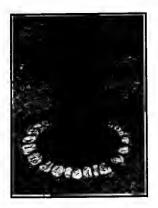
FIG 89. — Wall built around the base of a tree to prevent injury from earth filling. (See Fig. 88.)
