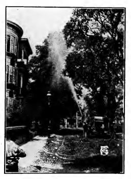
FIG. 107. — Spraying from the ground with solid stream and high pressure (Worthley nozzle).
