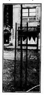
FIG. 59. - Effectual tree guard used on Boston Common. The wire guard is re-enforced by pointed angle irons driven into the ground.
