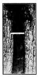
FIG. 56. — Chemically treated wooden block covering of cavity opening, with back re-enforcements of wood. The normal growth of the callus is not disturbed. (After J. A. Davis, City Forester, Springfield.)
