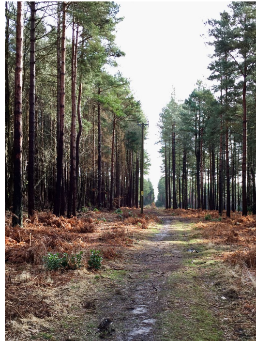
11kV power line
