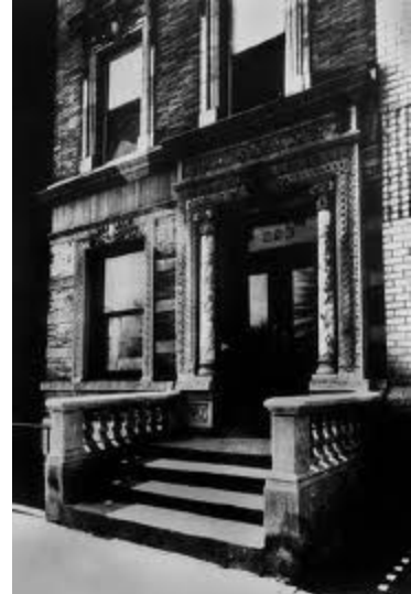
Towns Hospital 293 Central Park West
