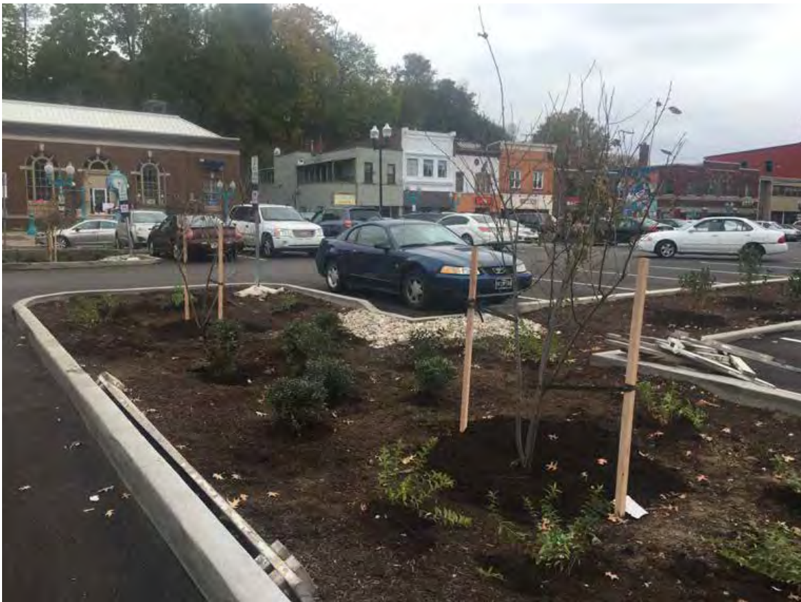
Rain gardens in renovated public parking lots, in Carnegie, PA, installed 2015.
