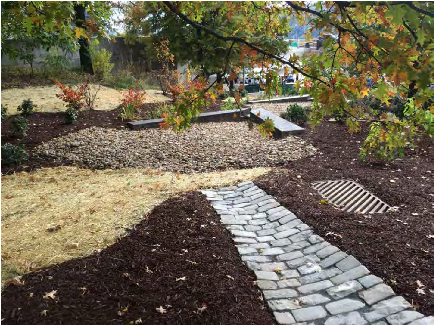
Bioswale at Point State Park, installed by WPC, 2015.
