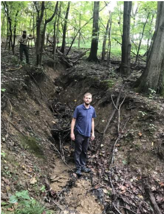
Severe Erosion Affecting Stream Morphology & Habitat.
