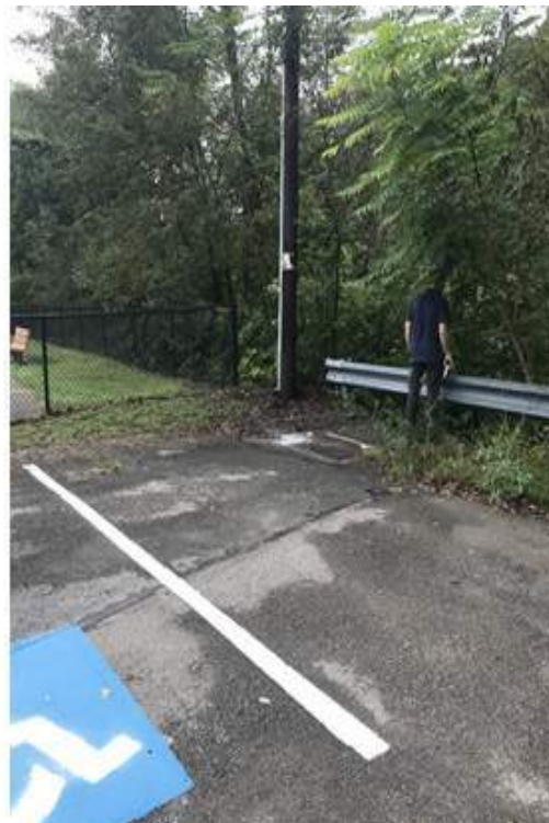
Parking Lot Catch Basin
