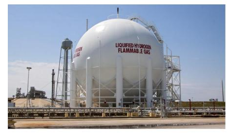
Figure 28: Liquid hydrogen storage vessel
