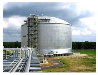
Figure 26: 15,000 tonne liquid ammonia tank Source: thyssenkrupp Uhde
