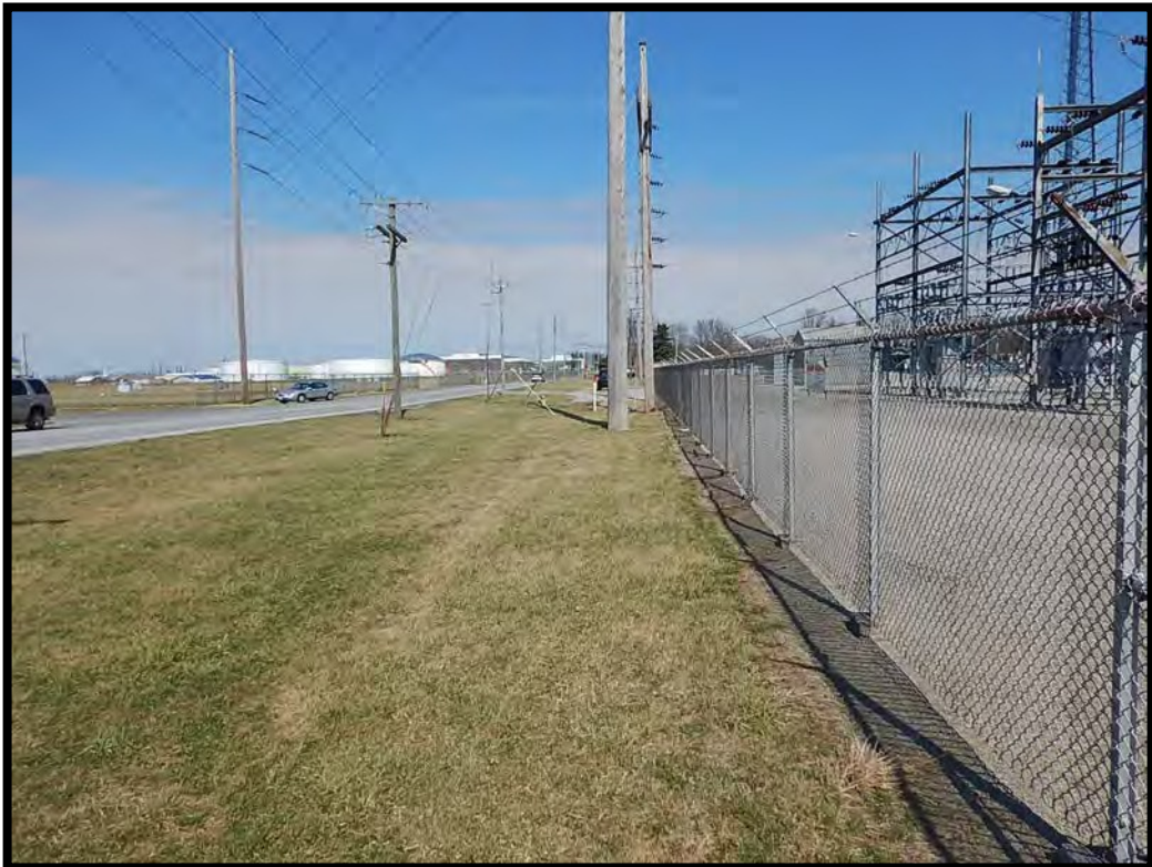
Figure 9. View of the disturbed conditions just east of McCain Rd.
