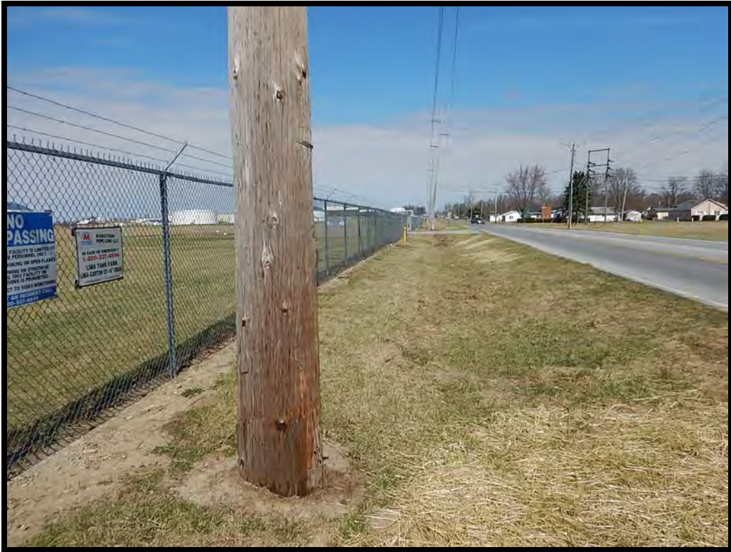
Figure 7. View of the disturbed conditions west of McClain Rd.
