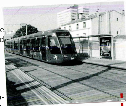
Montpellier's tram platforms are made of iron wood ( Tabebuia spp. ).
