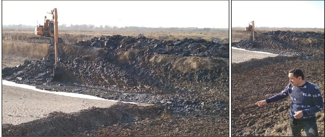
Figure 4. Excavation works in Otolikkol lake.
