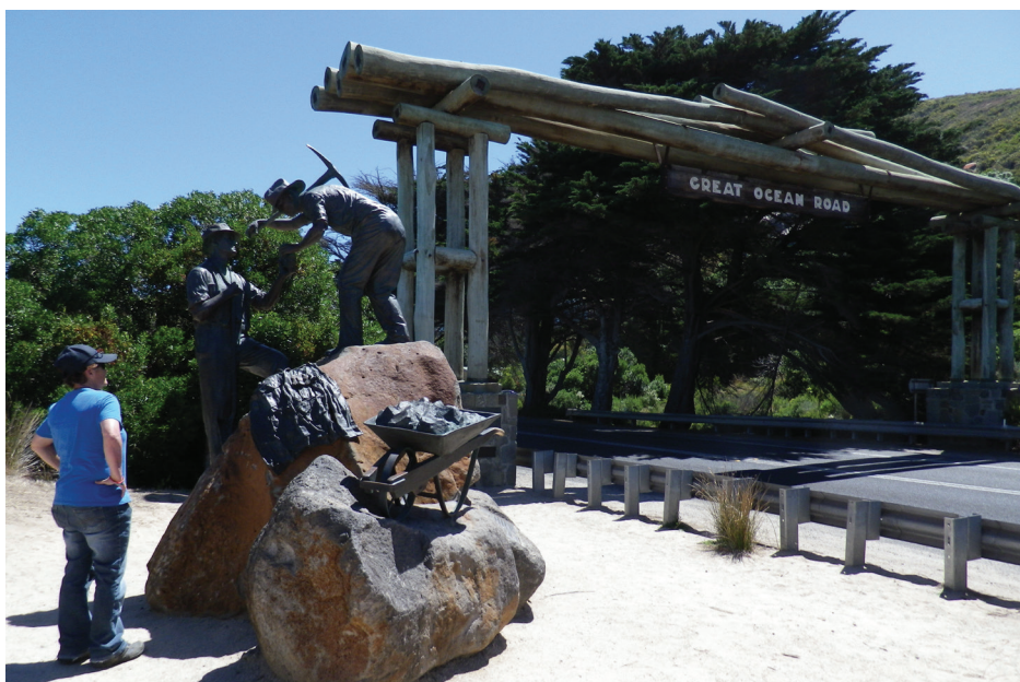
Figure 5.13 The Great Ocean Road is the only Victorian place of national heritage significance that includes areas of coastal reserve. This place also includes areas of road reserve and national park (Photo: M Mitchell)
