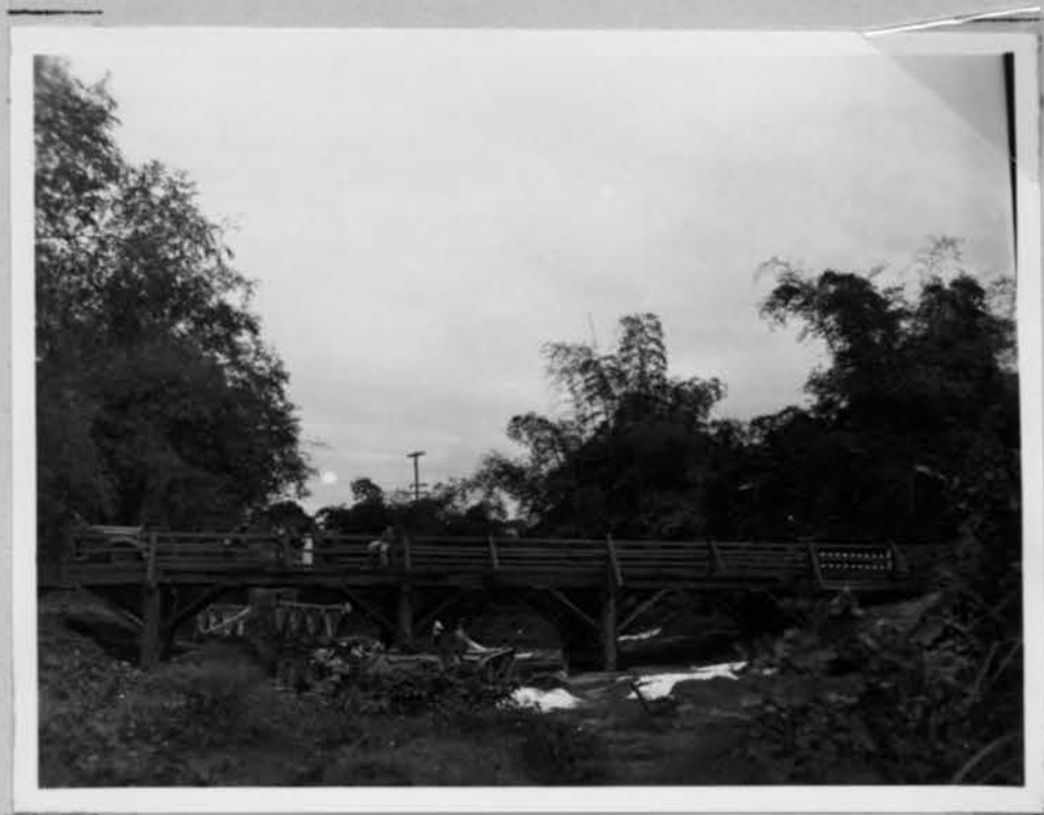
This bridge is typical of the many small, temporary bridges built by the Army.
