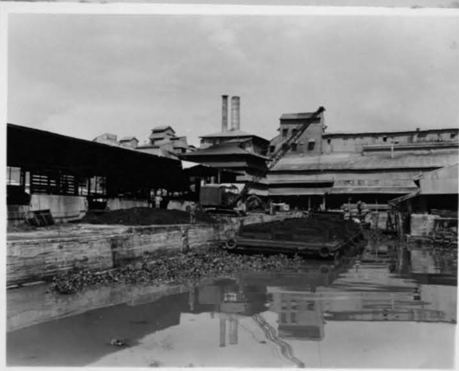
The cement factory at Binangonan, Laguna de Bay, Rizal Province. This factory suffered little damage and was put back into operation by the Army.
