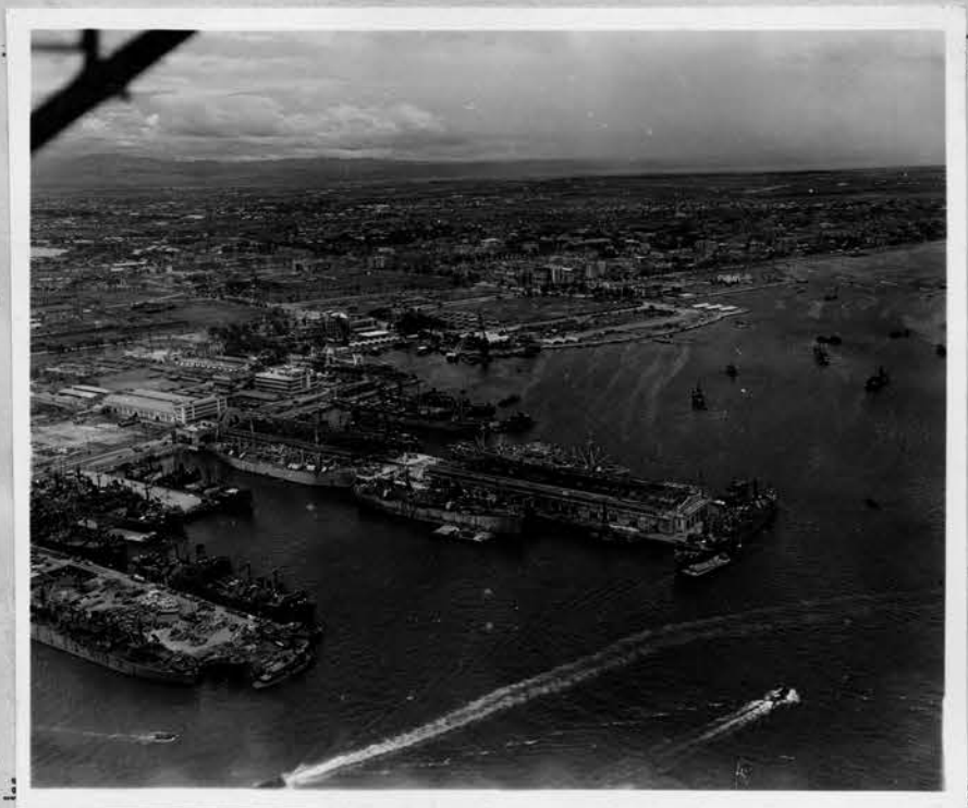
Pier #7, Manila. This is a pre-war pier that is still in operation after repair by the U.S. Army.
