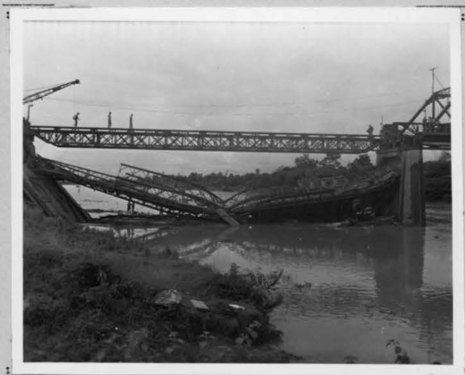
This bridge is part of the National Highway system and crosses the Mariquina River. Its repair was undertaken to serve the Army depots in the Mariquina River district.
