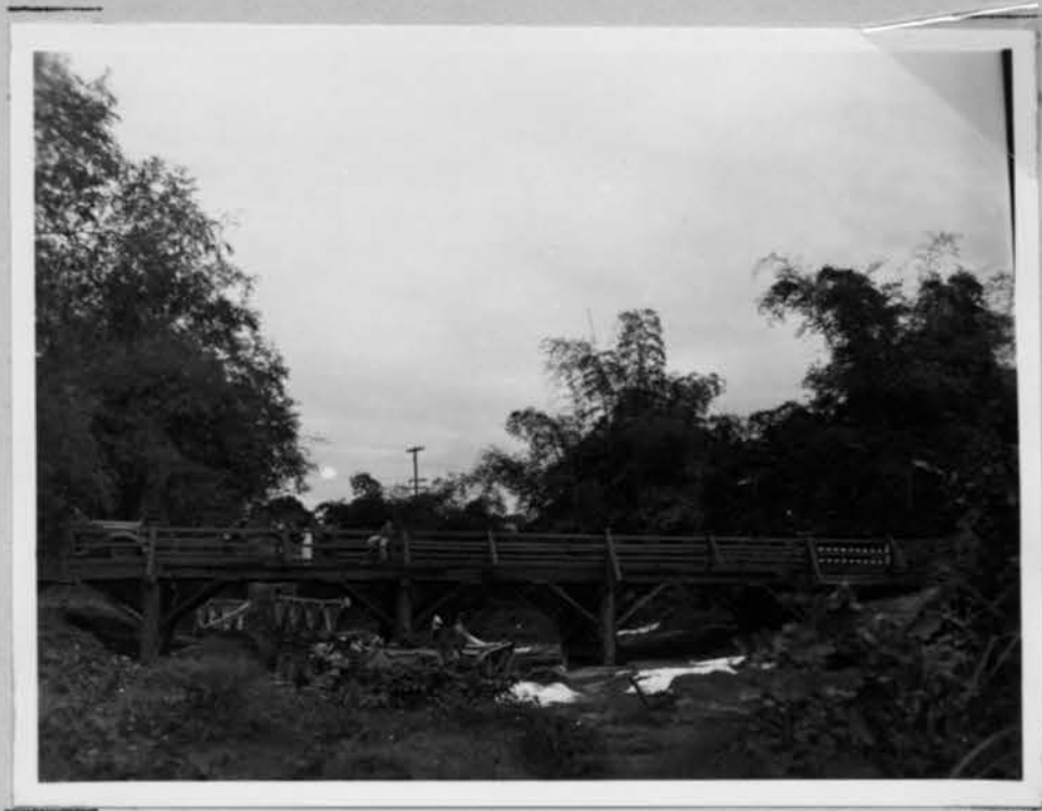
This bridge is typical of the many small, temporary bridges built by the Army.
