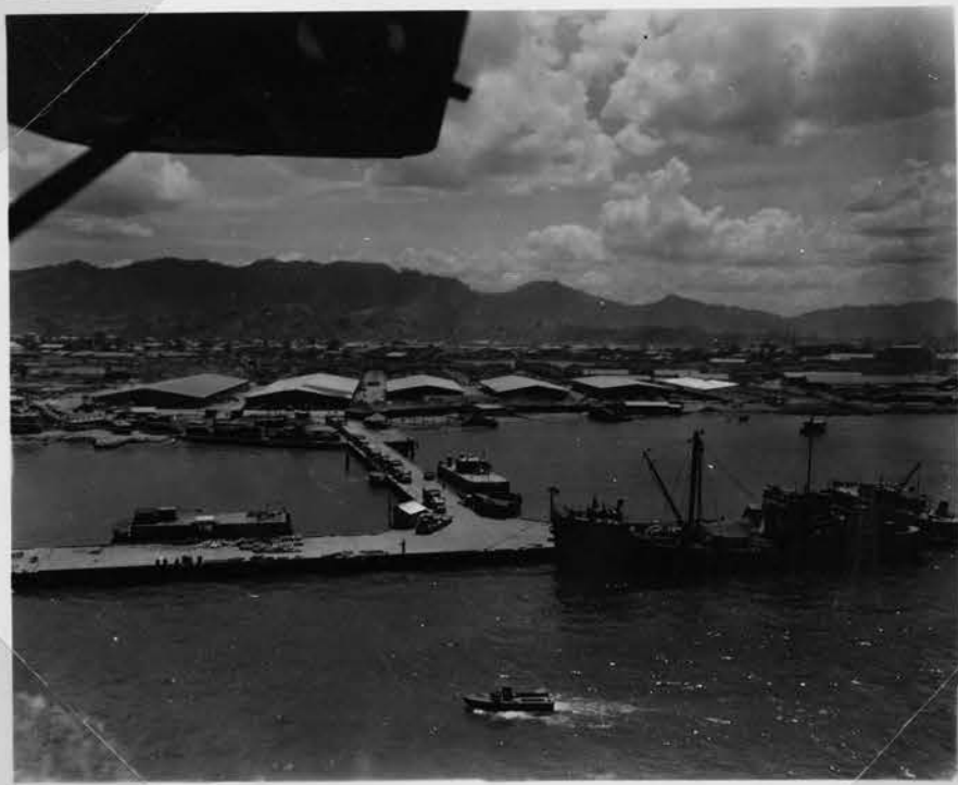
The Q.M. jetty at Base K, Tacloban, Leyte, P.I. Only shallow draft vessels of the F-S type are handled here.
