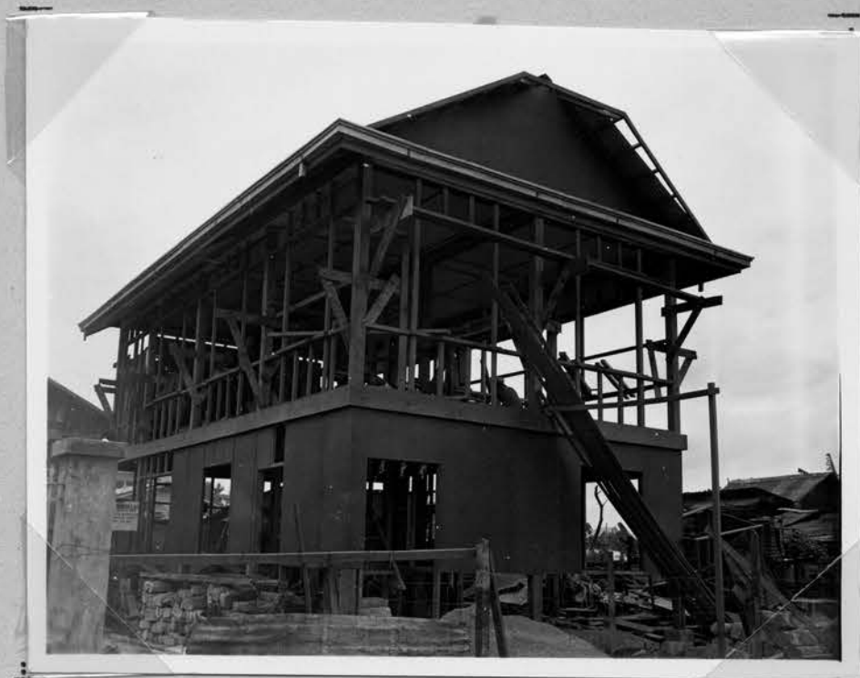
Those who are building new homes in the Philippines today say that it costs just about as much to build a 6 room house in the manner pictured as it used to cost to build a 12 room house of stone and tile. This house is of lumber and has a sheet iron roof.
