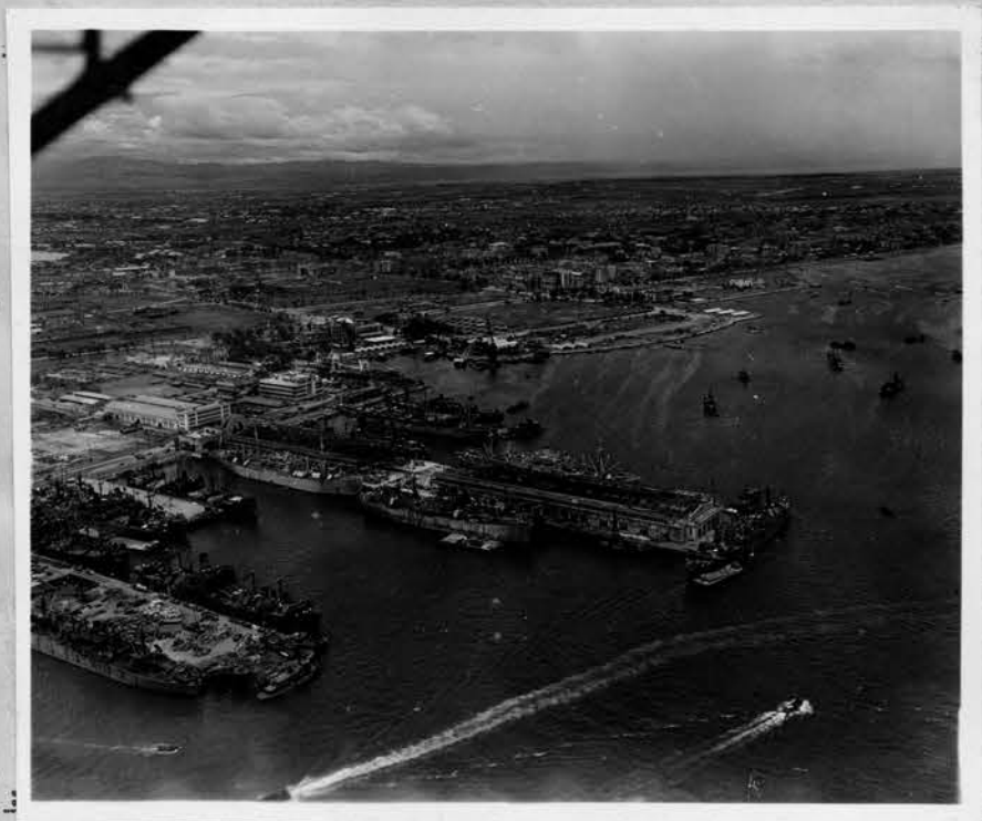
Pier #7, Manila. This is a pre-war pier that is still in operation after repair by the U.S. Army.
