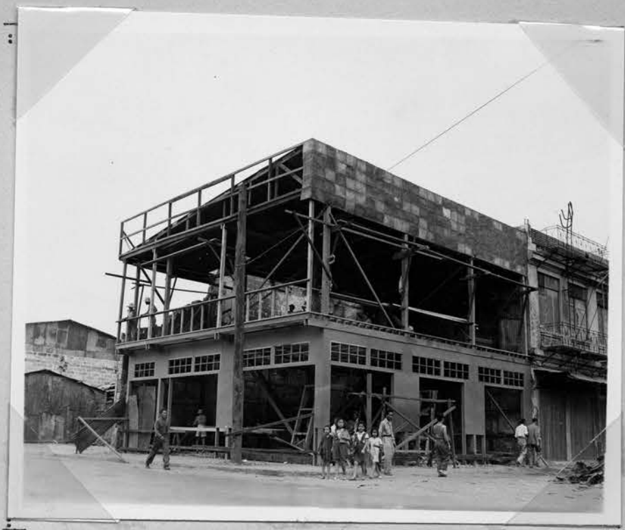
This building is typical of the flimsy, knocked-together sort of building which is going up in the Manila business district today. There is no steel, no concrete, no lumber, no glass in sufficient quantity to replace the great stone buildings that lined Juan Luna and the Escolta in pre-war Manila.
